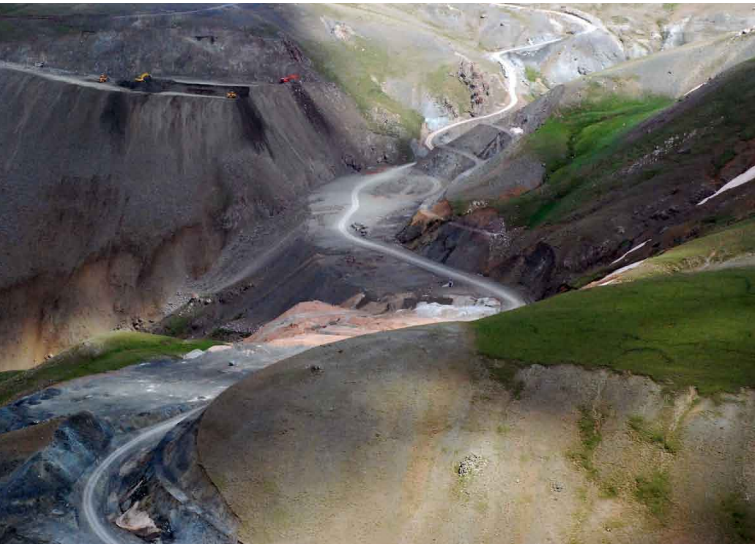
Road building, Palandöken Mountains PBA, Erzurum.
