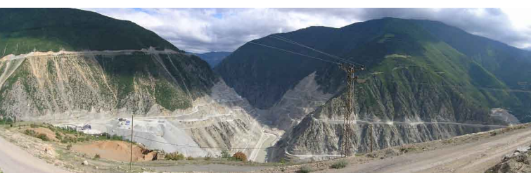
Artvin Dam under construction on the Çoruh River, Artvin.
