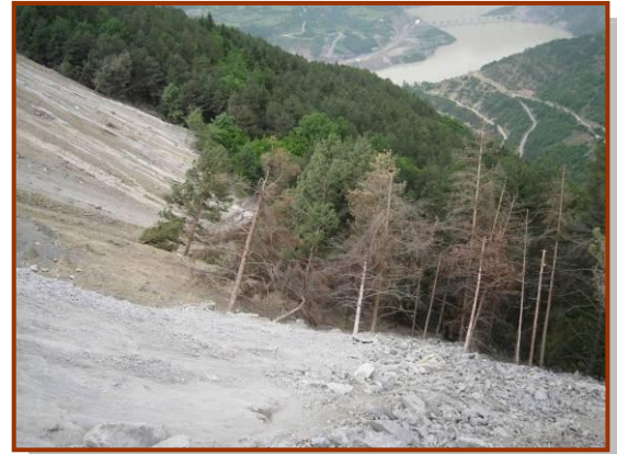
Construction debris pushed over the hill damages the slope vegetation. Photo Source: Oğuz Kurdoğlu
