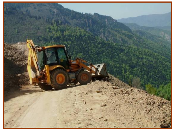
An excavator in the act of pushing debris downhill. Photo Source: Oğuz Kurdoğlu
